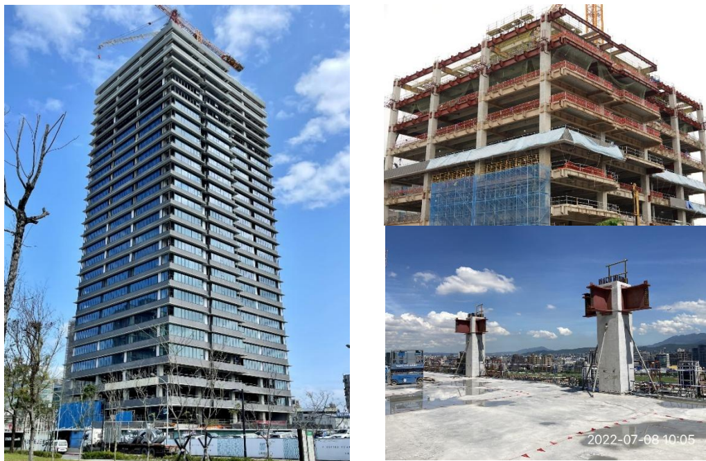
Fig. 19: View of the whole building and the typical steel-concrete MRCS connection detail.
